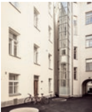
ELEVATOR INSTALLED OUTSIDE THE BUILDING IN AN EXTERNA SHAFT
