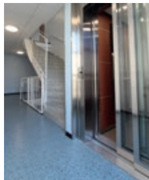
ELEVATOR INSTALLED NEXT THE STAIRWELL
