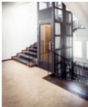
ELEVATOR INSTALLED INSIDE THE STAIRWELL
