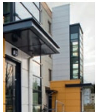
ELEVATOR INSTALLED INSIDE THE STAIRWELL, STAIRS MOVED OUTSIDE
